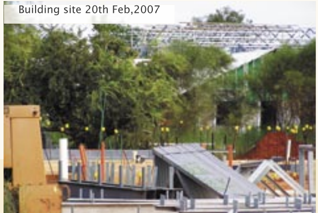
Building site 20th Feb, 2007
